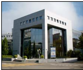
Nexus Telecom Zurich Headquarters
